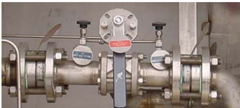
Rupture discs and crossover valve
