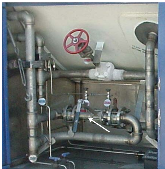
113C120W Dual Rupture Disc Assembly
