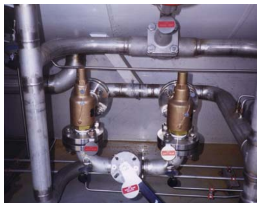
Dual pressure relief valve assembly
