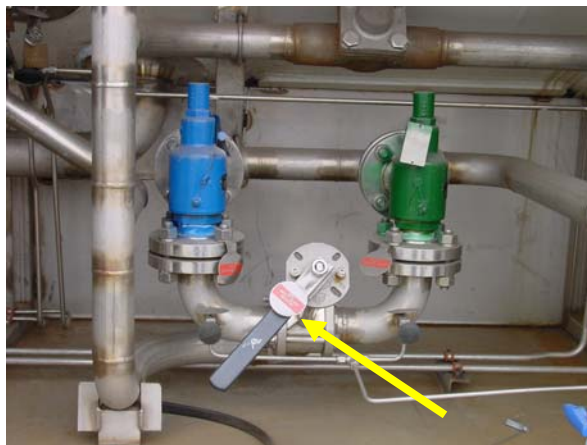
Pressure relief valve, with crossover (three-way) valve (arrow)
