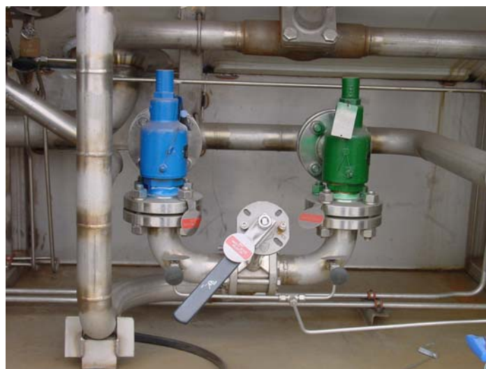
Pressure relief valves and crossover valve
